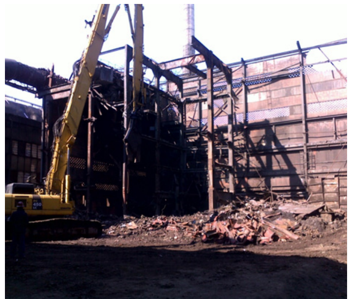
New FSF Site during demolition
