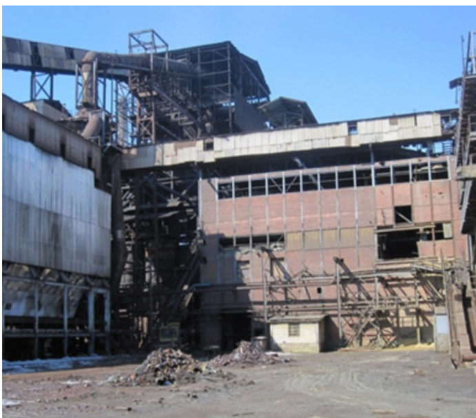
New FSF site prior to demolition
