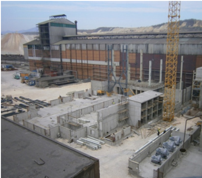
Construction Progress at 12/10/2012
